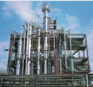
1993 DMC plant begins operation
