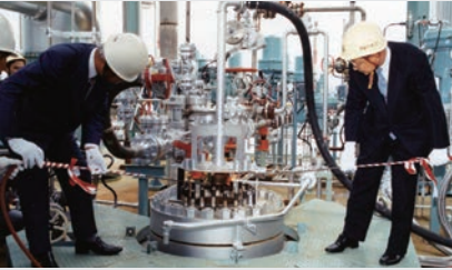
1984 Coal gasification plant firing ceremony
