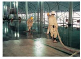
UBE's self-leveling material, Quick Ceramic Flow, being used at a construction site
